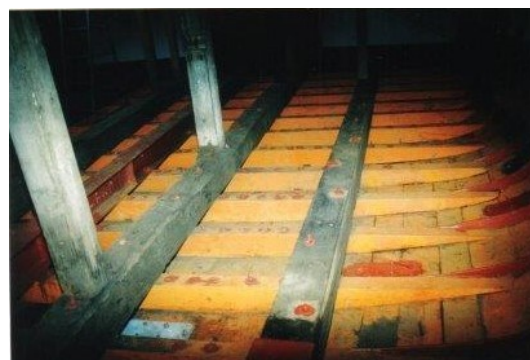
Oscar W after restoration showing floors all made by Malcolm.
