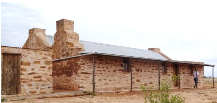
The restored Wilkins farmhouse at Mt Bryan East
