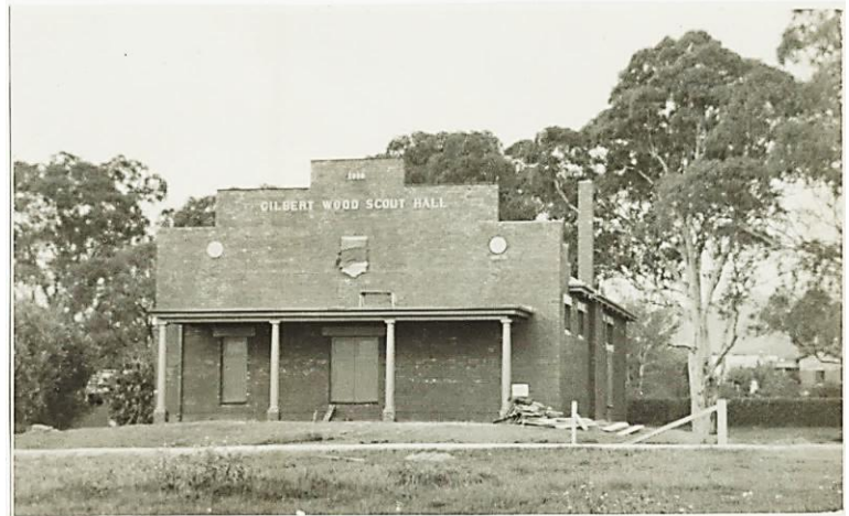
1st Linden Park Scout Hall [PRG 287/1/6/34] 1938. Note construction debris visible near the front verandah.
