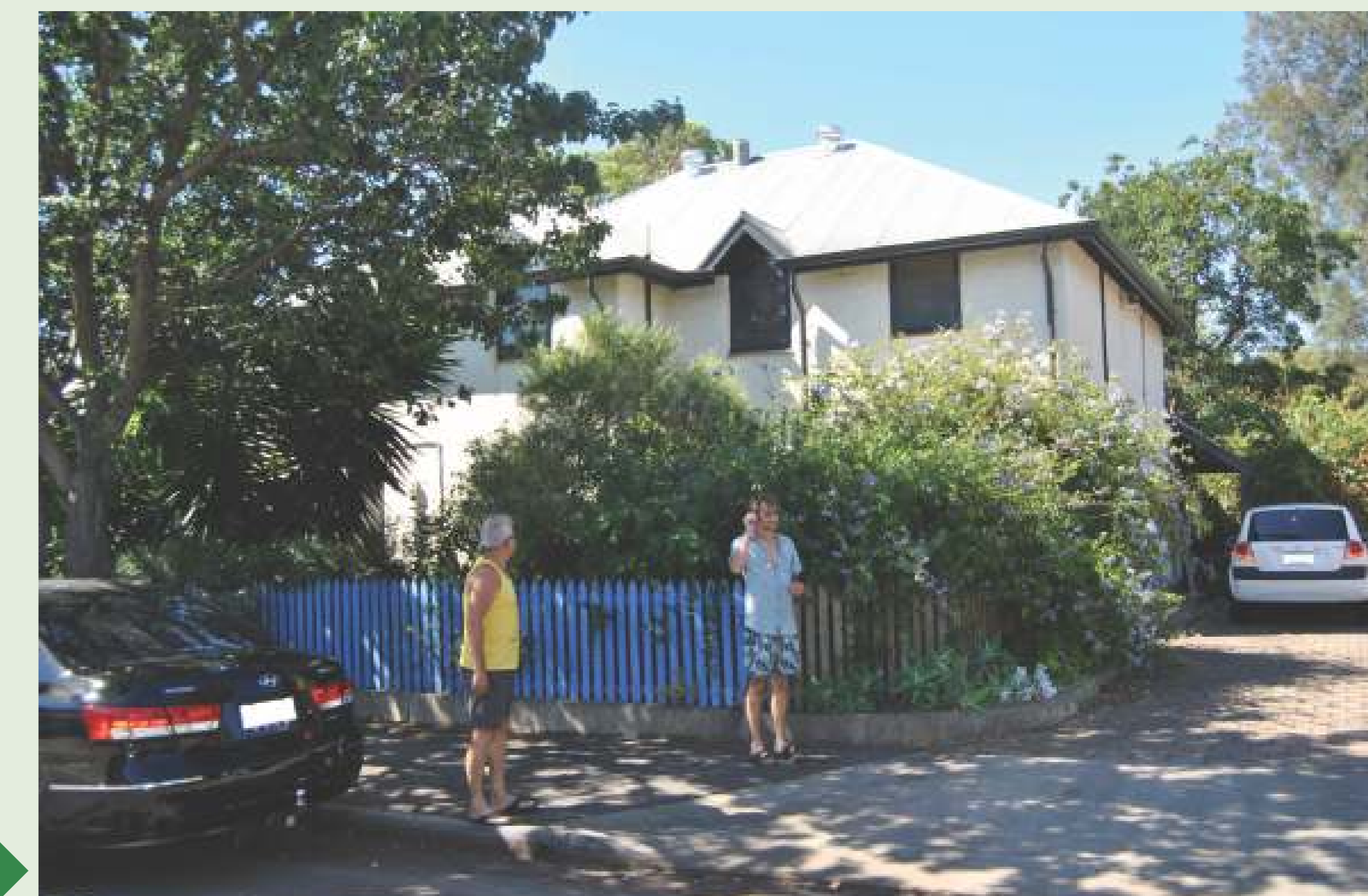
HHA earth built dwellings on Ninth Street, Bowden
