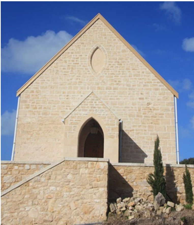
Image: Former Robe Bible Christian Chapel, 6 August 2013, showing north elevation with porch and reinstated blind gable opening. Source: Nominator
